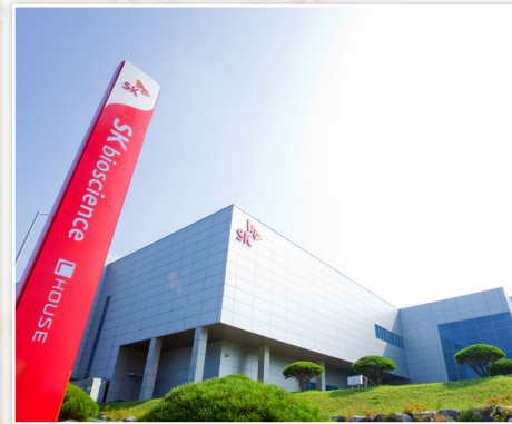
L HOUSE (Vaccine Manufacturing Plant)
