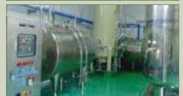
Improvement of Water Treatment Facility in Osan Plant
