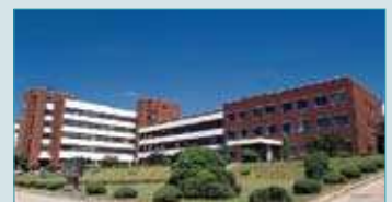
Former Research Center
