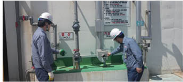
Checking hazardous chemical substance facilities
