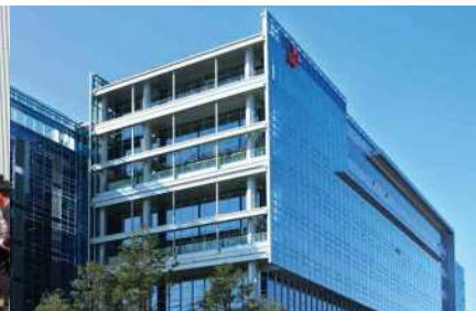
Completed building SK chemicals ECO Lab in September 2010
