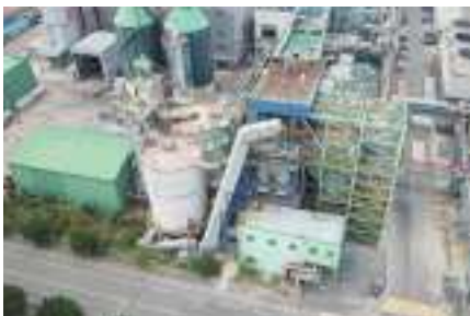
Eco Green Boiler(EGB)
